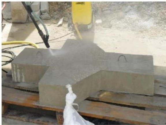
Figure 1: Surface Treatment by Sandblasting
