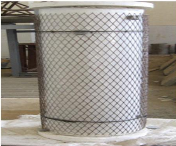
Figure 5. Steel in the form.
