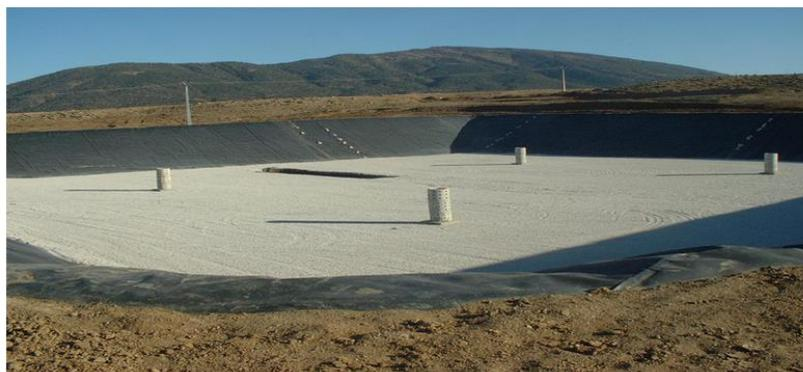
**Figure 1.** Landfill cell with biogas extraction chimney(*EPWG CET Constantine 2022*)
